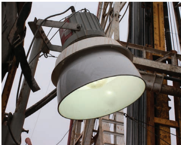
A 360 fixture fitted with one type of optional shielding.
