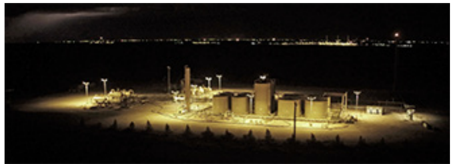
Apache Corporation tank battery using the latest dark sky friendly LED lighting technology. Note the light sources themselves are shielded from view, reducing glare, while providing a well lit working area. No light shines directly into the sky. Photo: Bill Wren/McDonald Observatory
