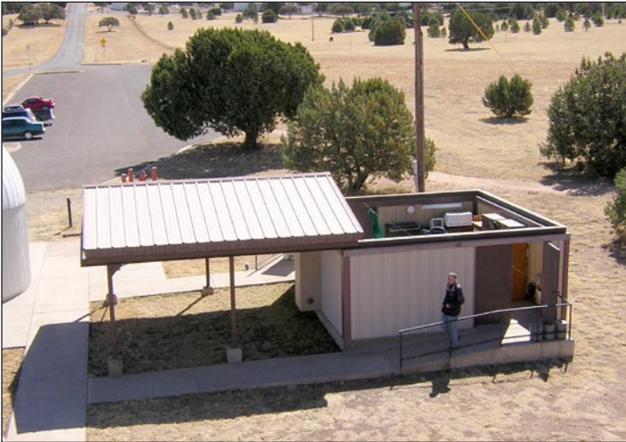
A roll-off roof observatory building gives an all sky view.
